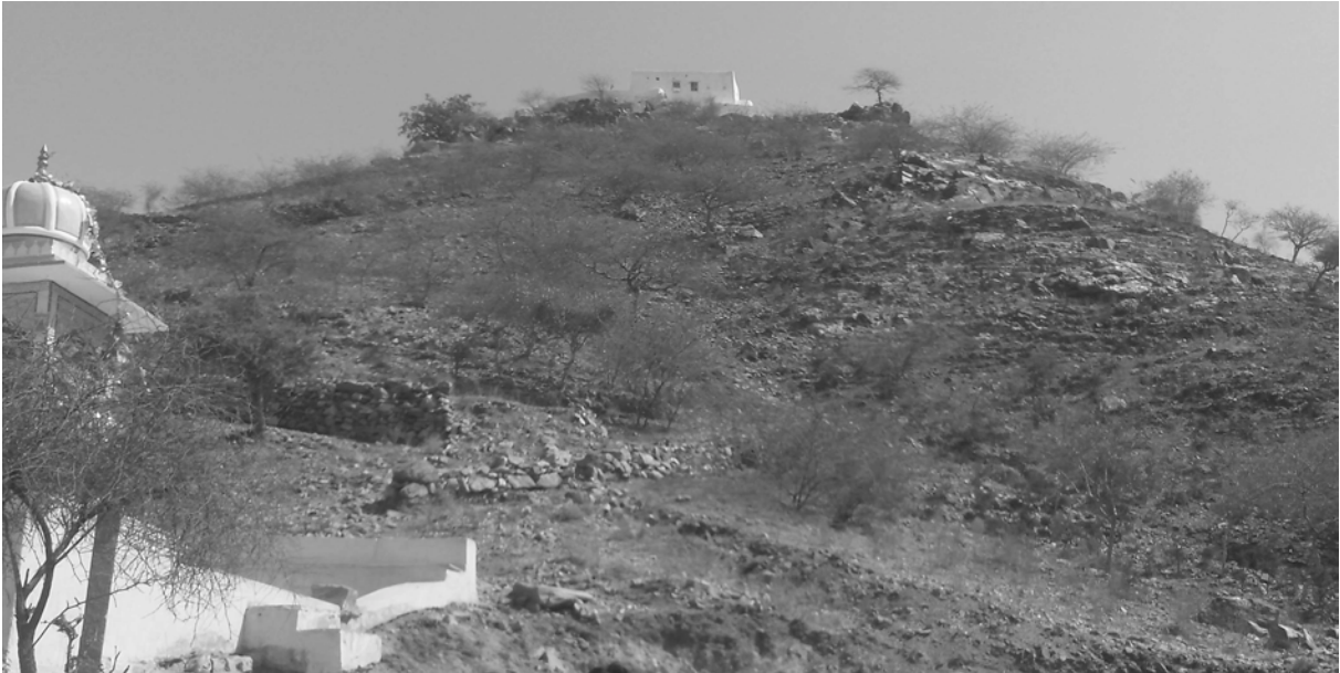
Fig. 3.1. Tikhi Dungari. The structure at the top is a samādhi built over the cave where Haridas is believed to have meditated for several years after being converted by Gorakhnath.
